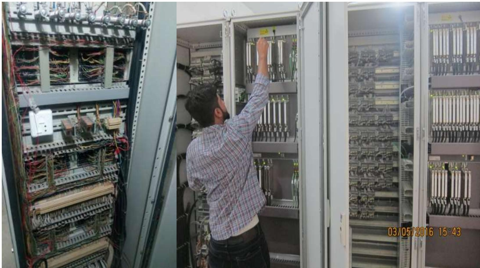
Old Signaling System replaced with Computer Based Interlocking Signaling System at Bin Qasim Station.
